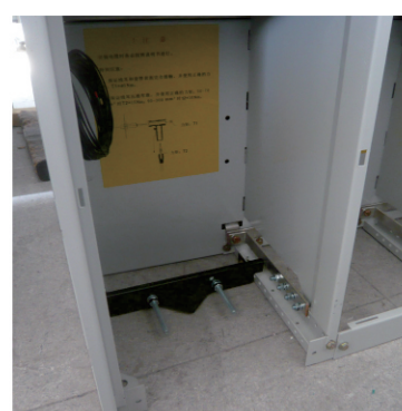
接地铜排 Ground copper bar
