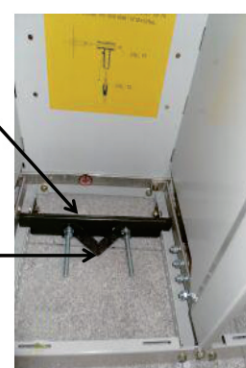
电缆夹梁 Cable clamped beam
