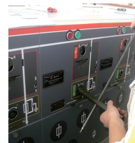
② 顺时针旋转操作手柄，闭合接地开关。 Rotate the operating handle clockwise to close the earthing switch
